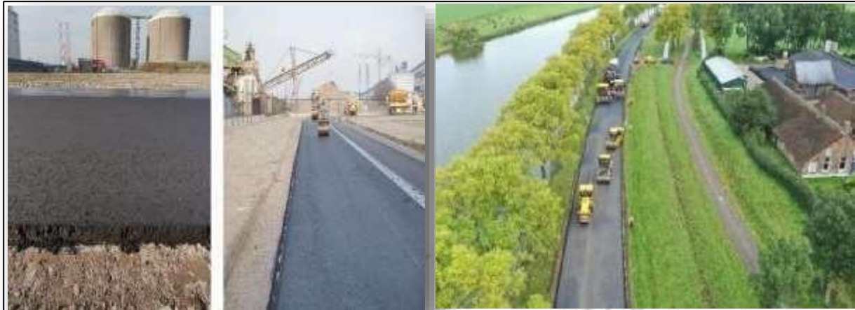
Figure 1: 12 km road stretch in Netherlands made with lignin (Source: Besamusca et al., 2021)
